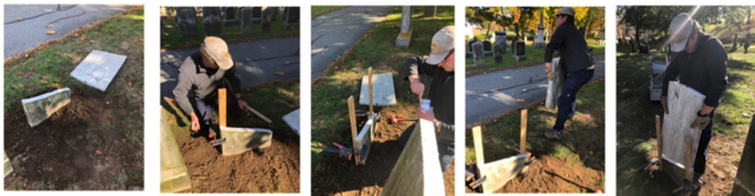
Repair of Angelina Gould Gravestone by Gravestone Services of New England (Kai Nalenz) October 22, 2022
